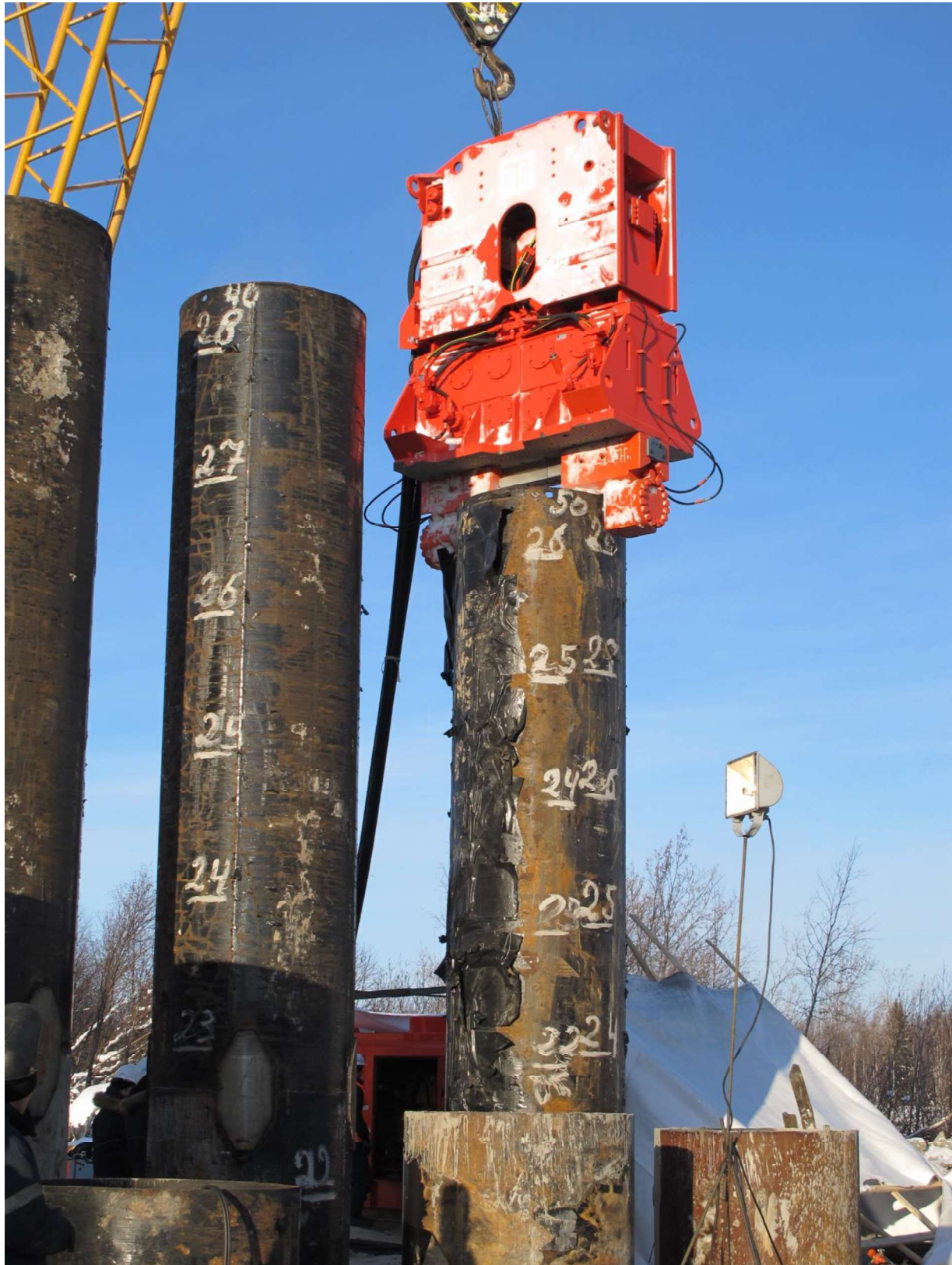
Sample photo of 120HD vibrator working with 2 x 150ton Duplex clamps:
